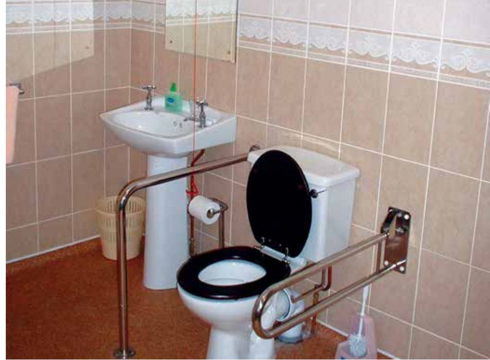
Bathroom with traditional fittings which contrast with walls and floor
